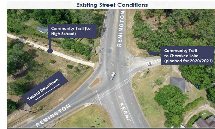
Remington, Reid and Kern Intersection
