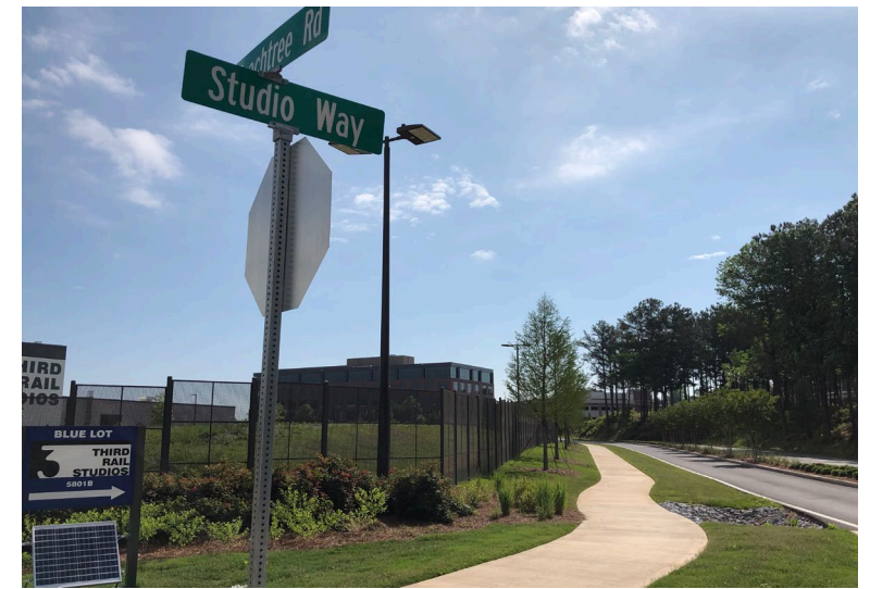
Assembly CID Road and Utility Infrastructure Phase I 5 th Round (June 2017)
